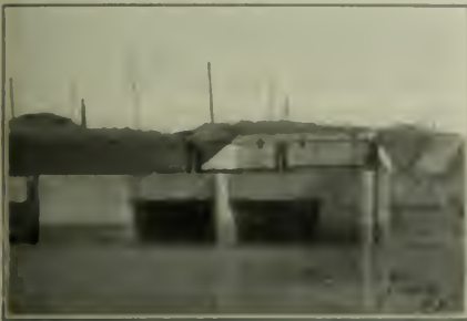
MOUTH OF INTAKE TUNNEL
